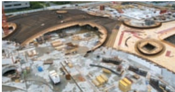
Big shell formwork. Photo courtesy of designtoproduction
