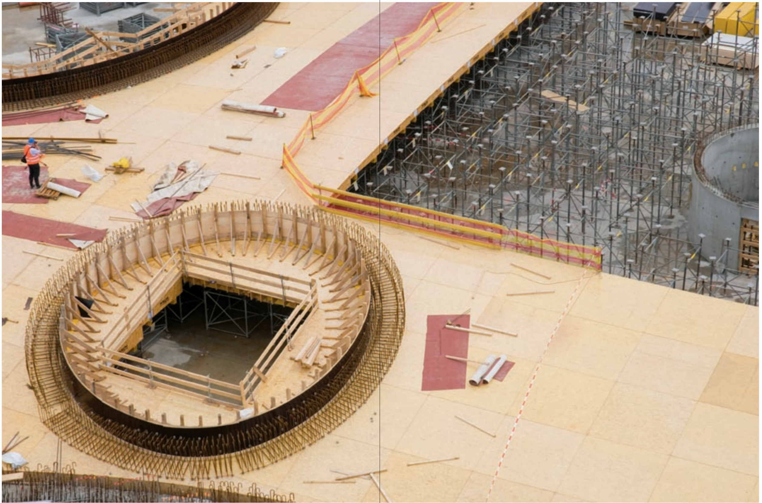
Big shell formwork. EPFL learning center, Lausanne. Photo courtesy designtoproduction
