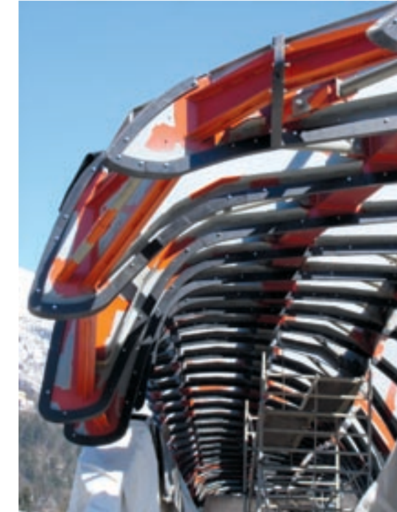
Hungerburg Funicular, Innsbruck, Austria, Zaha Hadid, 2006. Profiles mounted to the steel sections of Lowenhaus Station. Photo courtesy of design to production
